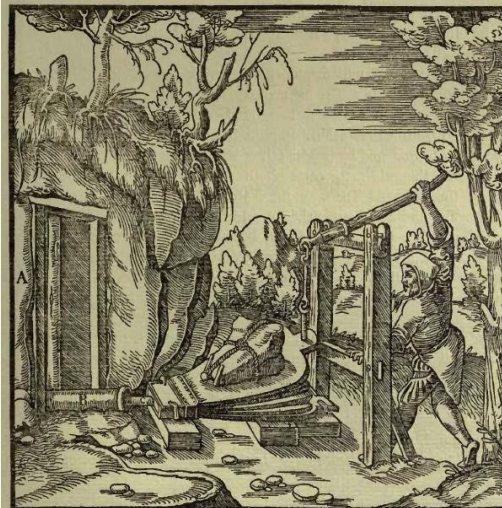
A—TUNNEL. B—PIPE. C—NOZZLE OF DOUBLE BELLOWS.
