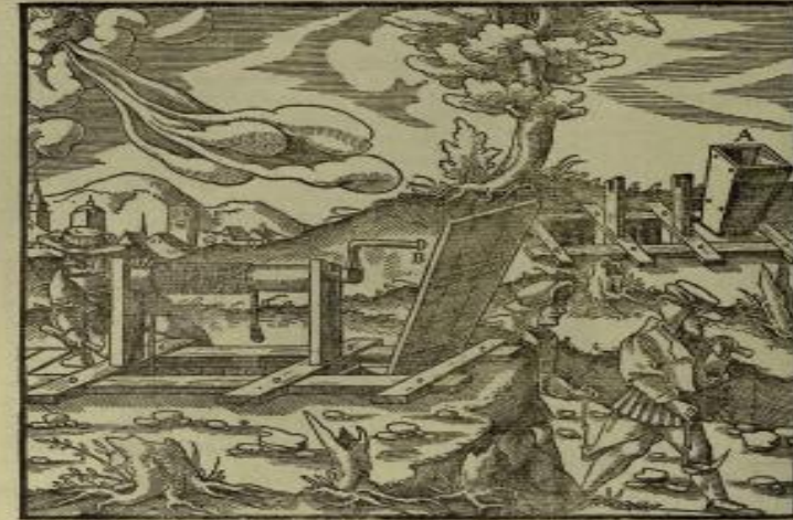
A—PROJECTING MOUTH OF CONDUIT. B—PLANKS TIED TO THE NORTH OF THE CONDUIT WHICH DOES NOT PROJECT.
